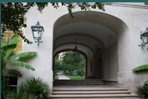
The IES is centrally located in Upham Hall
